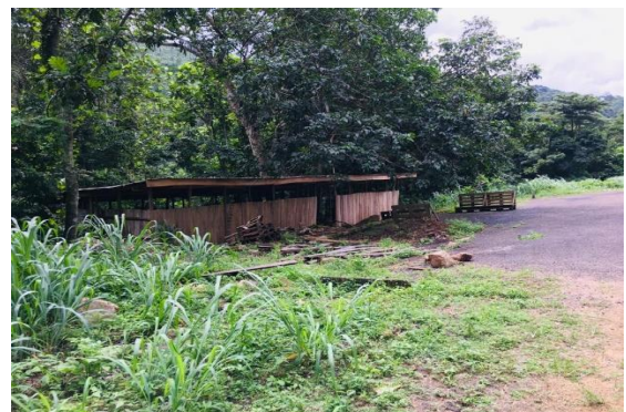
Figure 16: Plates 16 - Dilapidated shed for relaxation
