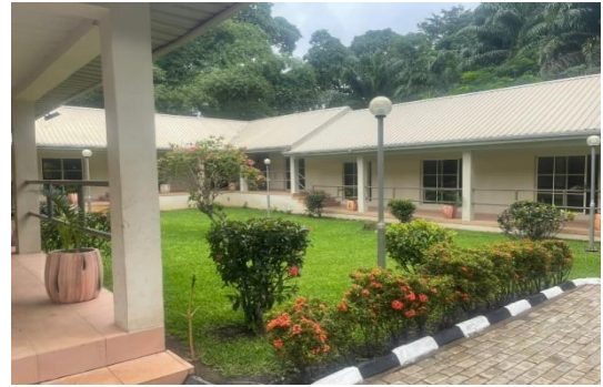
Figure 4: Plate 4 - A part of the chalets for accommodation
