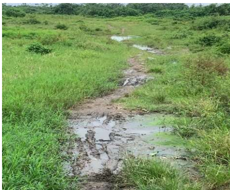
Plate 3: Deplorable Road of Emirin dumpsite
